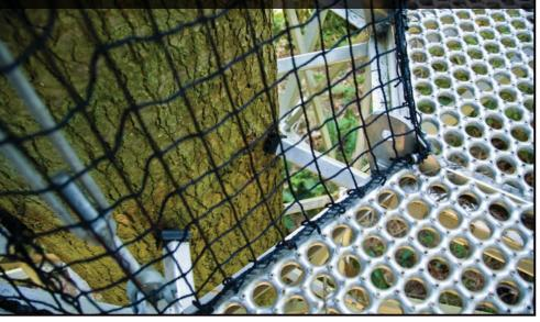
The Greenheart Conservation Company constructed the walkway using "Treehugger" technology, a system of interlaced steel cables that keeps the trees unharmed; neither nails nor bolts have to be used to attach spans and platforms. This Canadian company constructs nature-based attractions, including walkways and flightlines, all around the world, capitalizing on the popularity of eco-tourism—and there's nowhere greener than Vancouver.
