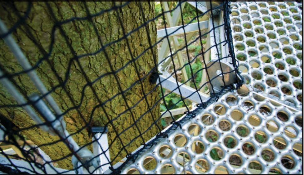
The Greenheart Conservation Company constructed the walkway using “Treehugger” technology, a system of interlaced steel cables that keeps the trees unharmed; neither nails nor bolts have to be used to attach spans and platforms. This Canadian company constructs nature-based attractions, including walkways and flightlines, all around the world, capitalizing on the popularity of eco-tourism—and there’s nowhere greener than Vancouver.
